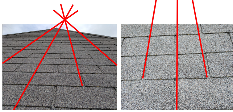
Figure 3.4: Left - Non-orthogonal imagery with single-point perspective. Right - As the vantage point moves toward an orthogonal position, the perspective is reduced.
